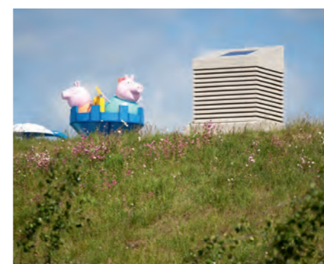
■ Seven windcatchers protruding from the rooftop reveal the building's self-ventilation system
